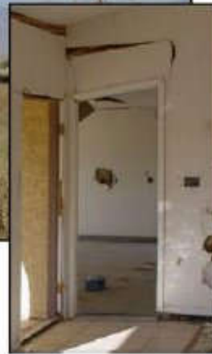
Fig. 8 - Earth fissure damage to residence in Nevada (photo by John Bell)
