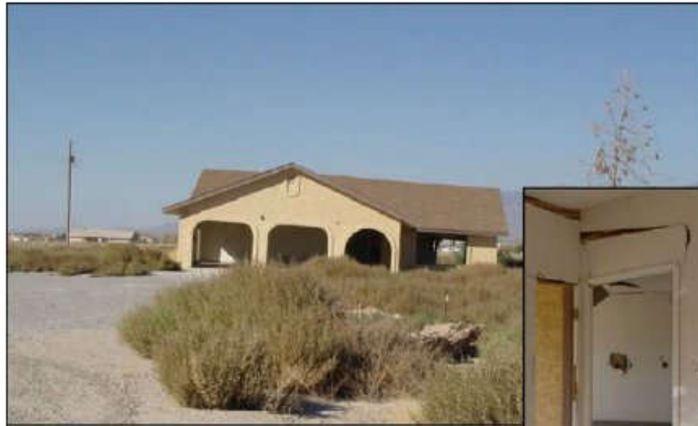
Fig. 8 - Earth fissure damage to residence in Nevada (photo by John Bell)
